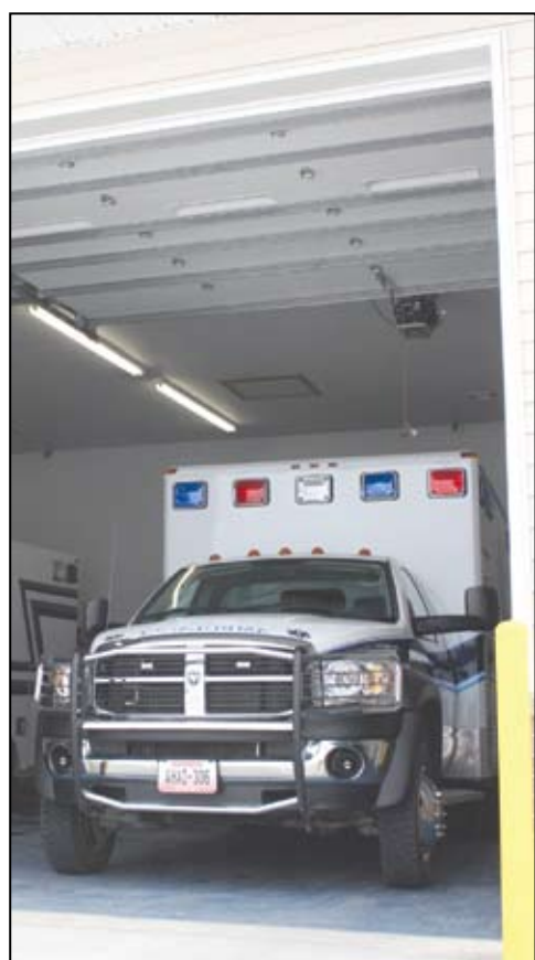
The new ambulance bays- Provide ample room for the larger Dodge-based ambulance and much easier access to each vehicle when emergencies arise.
