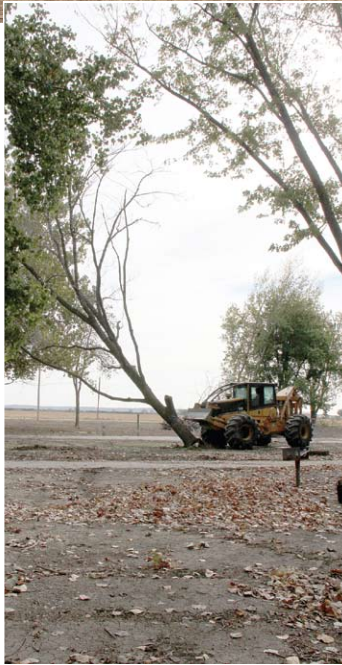
Logger Gary Greene- Pushed over another tree in the campground area at Big Lake State Park. The job of removing so many trees was a difficult task as Greene had to dodge many obstacles. The picture is taken from the lake side, making obvious the different landscape change looking to the east toward the highway. Previously, the highway was not easily visible through the trees.
