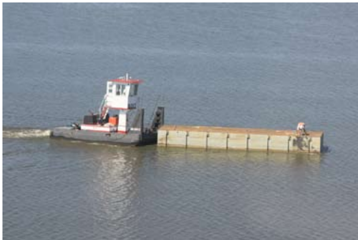
"You know if you see a tugboat in your field----- You've got PROBLEMS!!" This tugboat was pushing part of a section barge to the worksite of the Burlington Northern Santa Fe railroad west of Fortescue, MO. The section barge will be used for the work being done by Massman Construction to construct a 200' trestle railroad bridge at the site.
