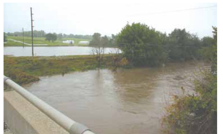
Water levels at Squaw Creek National Wildlife Refuge - Rise over the banks on Wednesday, Sept. 10. According to a release by the Missouri Department of Conservation, swollen refuge waters flooded nearby roads following the Tuesday, Sept. 9, storm.
